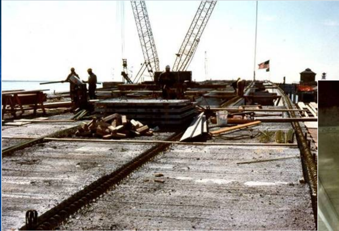
Precast deck slab placement
