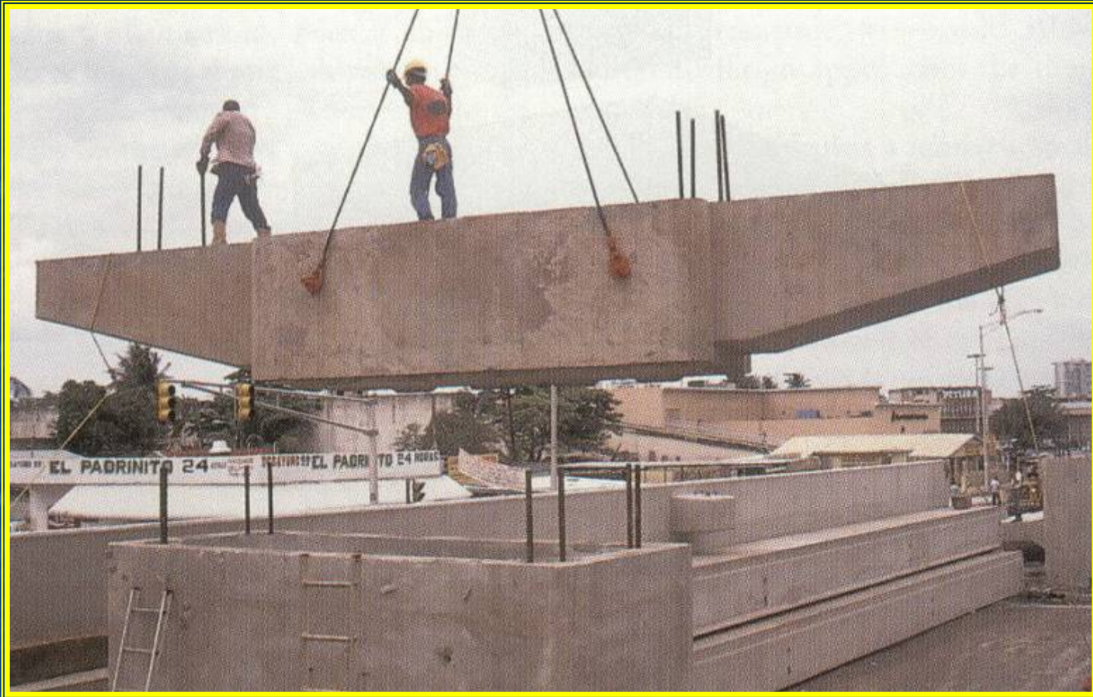
Precast pier cap installation
