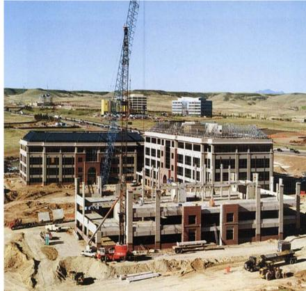
Structural and architectural precast components used in the CH2M Hill project accounted for 39 percent of the materials used to calculate the local/regional content of the buildings.
