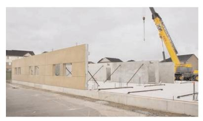
Exterior walls were insulated sandwich wall panels with a two tone sandblasted exterior finish. Ledges were provided on the back of the load bearing panels to support the hollow core roof slabs.
