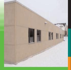
The project consists of a new self contained 1020 sq m (11,000 sq ft) addition consisting of 10 classroom plus toilets and a teacher's room that is directly connected to the existing school. All of the structural components above the foundations were precast ahead of time and delivered to the site for fast installation:
