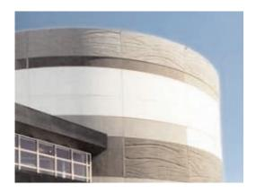
"Precast concrete was selected because it fully met the requirements of the LEED program," states Alain. "Durable, fireproof and recyclable, this material helps obtain superior energy efficiency. It makes it possible to obtain flawless soundproofing, an important feature, particularly in the case of a concert hall such as the one in the new pavilion."
