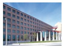
tight control on the concrete mixing process as well as sandblasting the panel surfaces gave the building the appearance (colour and texture) sought. The panels achieved the goal set out - the architectural beauty of precast concrete.
