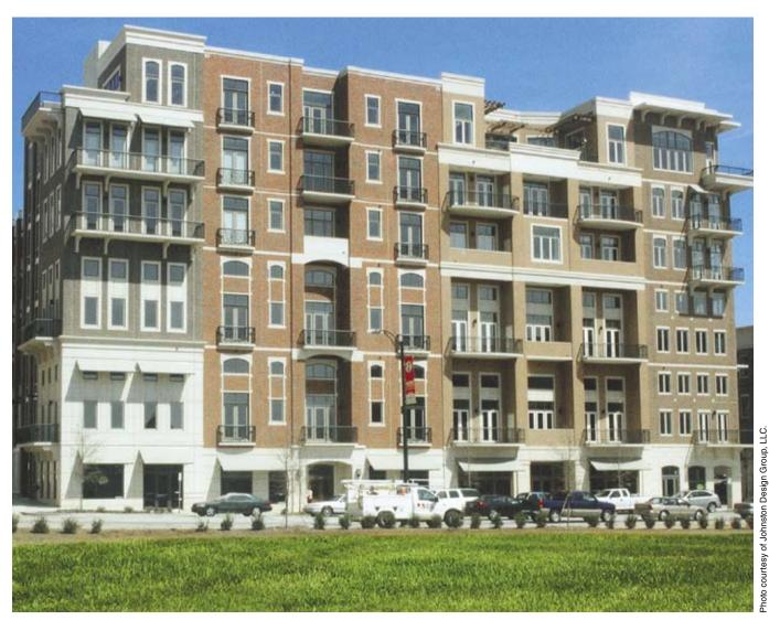
**Fig. 3**. A U.S. Green Building Council (USGBC) LEED-registered, mixed-use development, the "Bookends" in Greenville, S.C., features street-level retail and residential condominiums. The precast concrete walls have a combination of sandblasted and cast-in thin brick finishes. The facade of this building has four distinct architectural styles to appear as four separate and unique buildings.
