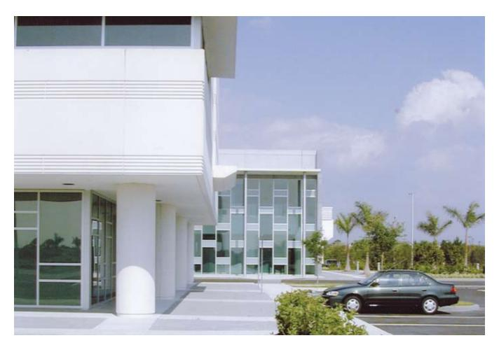
**Fig. 4**. In cities such as Cape Coral, Fla., mitigating the heat island effect is especially important. Note the white color of the architectural precast concrete—built for the city of Cape Coral City Hall.
