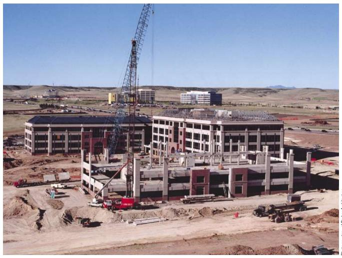
**Fig. 1**. The buildings in the corporate campus for CH2M Hill in Englewood, Colo., are framed with a total precast concrete system, including precast shear walls, double tees, inverted tee beams, and load-bearing exterior walls. The buildings are some of the first Leadership in Energy and Environmental Design (LEED)—certified total precast office buildings.
