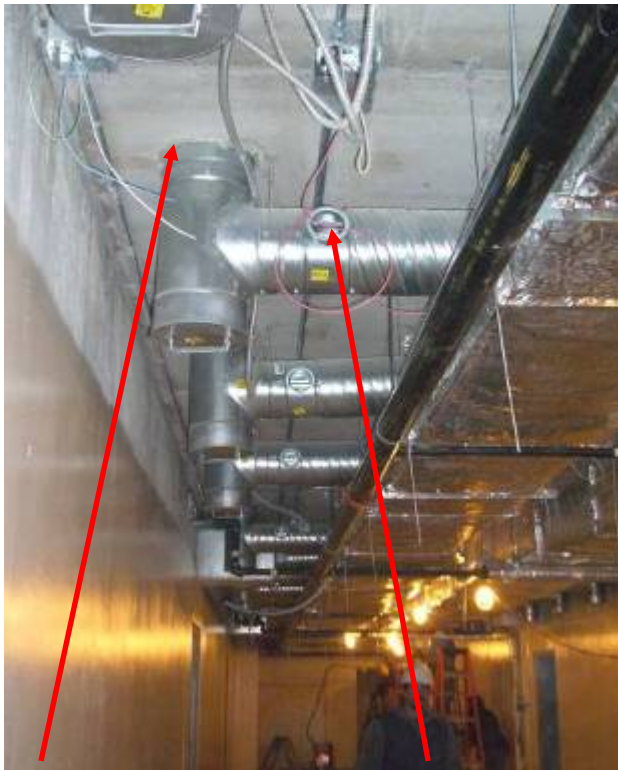
Connection to the Slab Balancing Damper (Typical)
