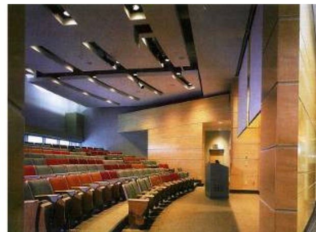
40% Openings In Suspended Ceilings
