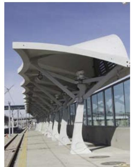
Fig. 10. Site constraints, above and below grade, restricted the width of the platform, minimizing the overall LRT Station footprint. This walk-on station is designed as a side-loading platform, staggered to improve passenger safety across the tracks. (Courtesy of Lafarge.)
