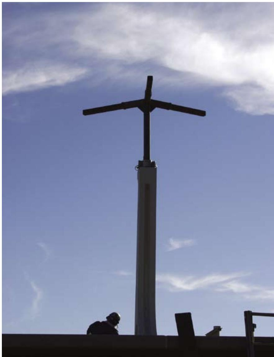
Fig. 19. Three-legged assembly cross on each column provided an anchor for hoisting the struts into place. (Courtesy of Lafarge.)
