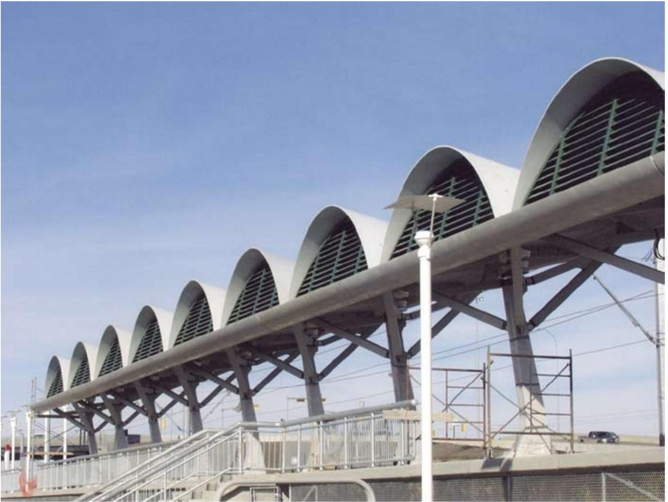
Fig. 9. Repetition of form provided formwork, precast concrete production, and erection economies. (Courtesy of Lafarge.)
