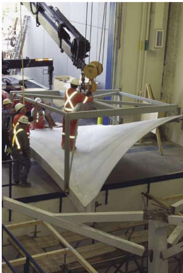
Fig. 15. Installation of the prototype canopy at the University of Calgary's Centre for Innovative Technology. (Courtesy of Lafarge.)
