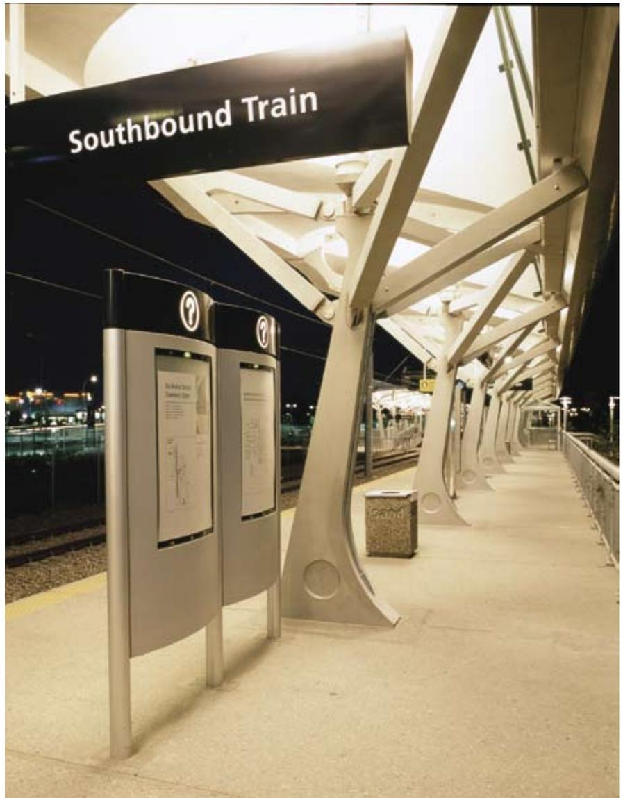
Fig. 2. Night-time photo of the Shawnessy Light Rail Transit (LRT) Station in Calgary, Alberta, illustrates the commuter-friendly ambience and durable function of a novel UHPFRC design. (Courtesy of Tucker Photo.)
