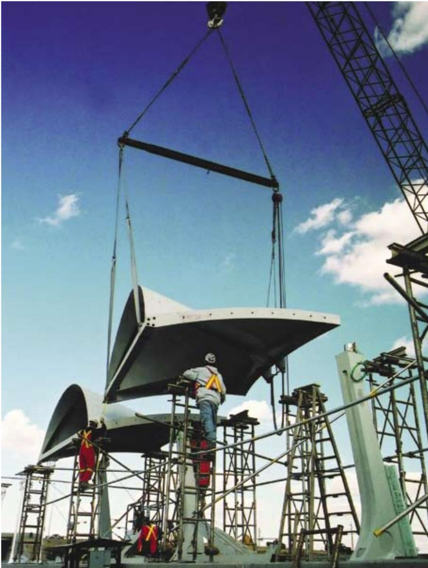
Fig. 21. Crane set of canopy over assembly cross. Note chain hoist for lifting struts into position. (Courtesy of Lafarge.)
