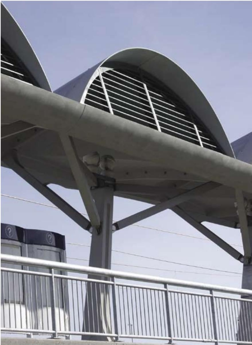
Fig. 8. A single, slender column gracefully supports each precast concrete shell and serves as a conduit for communication, security, and electrical cabling. (Courtesy of Lafarge.)
