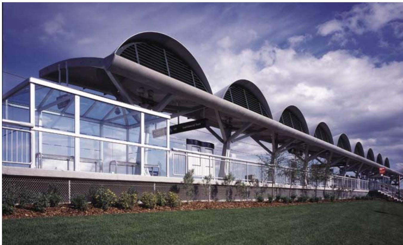
Fig. 7. Thin, graceful precast concrete shells provide an uplifting and airy ambience for commuters. (Courtesy of Tucker Photo.)
