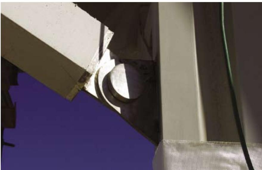
Fig. 22. Strut to mid-column connection. (Courtesy of Lafarge.)
