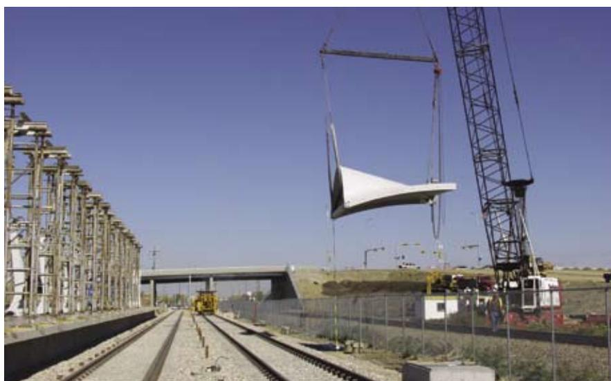
Fig. 20. Crane hoists thin-shell canopy over rapid transit rail lines to assembly frame. (Courtesy of Lafarge.)
