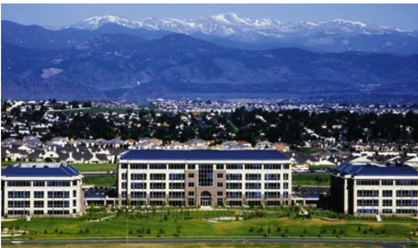
Mahogany-colored precast accentuates the buildings' bases and entries. Both the mahogany panels and the limestone field panels were acid etched. The three buildings are joined by an enclosed ground-floor passage.
