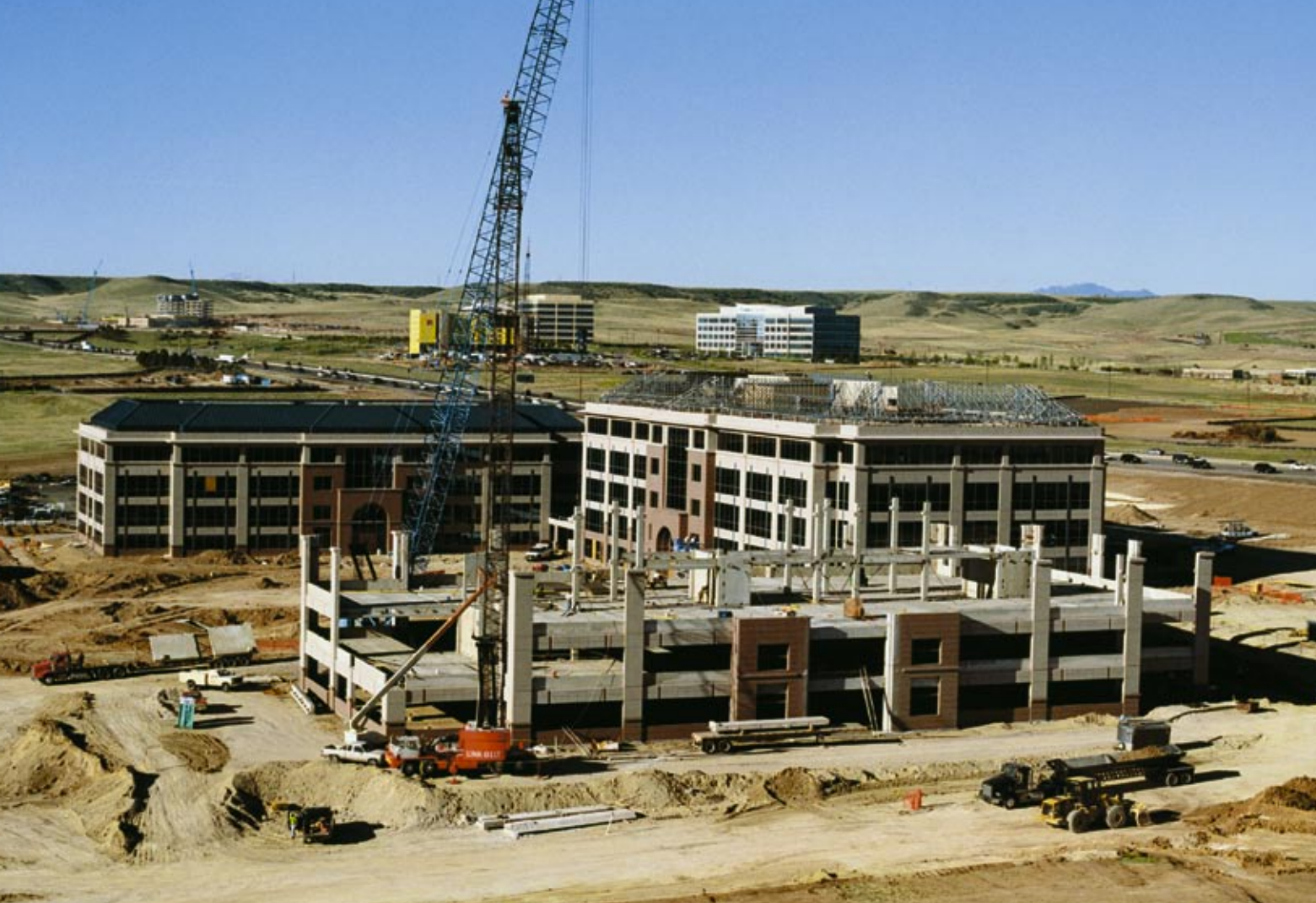
All three buildings feature total-precast structural systems. The third building, in the foreground, is a support structure that houses the data center. It was designed, fabricated and erected in just 11 months. Rocky Mountain Prestress was both the precaster and the erector.
