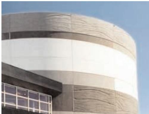
"Precast concrete was selected because it fully met the requirements of the LEED program," states Alain. "Durable, fireproof and recyclable, this material helps obtain superior energy efficiency. It makes it possible to obtain flawless soundproofing, an important feature, particularly in the case of a concert hall such as the one in the new pavilion."
