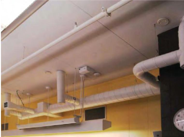
TermoDeck in combination with hollow core slabs can create an environmentally sound building, with an extremely efficient, cost-effective method of heating and cooling. This method also provides the added benefits of improved indoor air quality, ventilation, and comfort by constantly importing fresh, clean air into the building and exhausting old, stale air.
