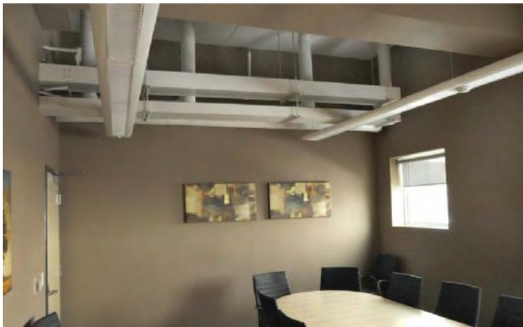
heating and cooling system developed in Sweden. TermoDeck uses hollow core concrete slabs to distribute air that takes advantage of the thermal mass of the building for heating and cooling. Up to 70% of the heating or cooling of rooms is accomplished by radiation, directly heating or cooling the occupants with the stored thermal mass, rather than conditioning the air around them.
