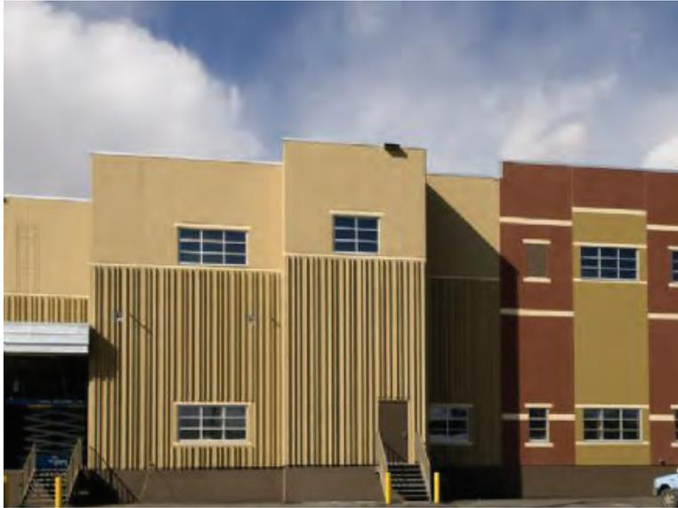
Dow Chemical PANELMATE™ with a thickness of 4 inches which provides an R value of 21 in the panel system.
