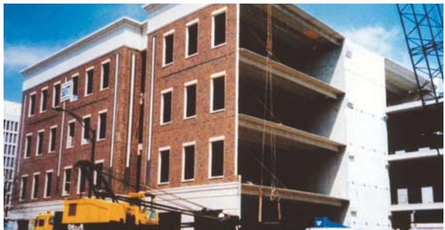
NBSC Headquarters building (opposite page) in Greenville, S.C., was converted to a total precast structure from its original design of structural steel with a brick veneer. The load-bearing precast panels (above) have cast-in brick units and sandblasted precast sills and headers around the precast openings.
